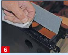
Cut to size and then apply foam (included in the kit) to the outer flap by pulling back the protective cover as shown
